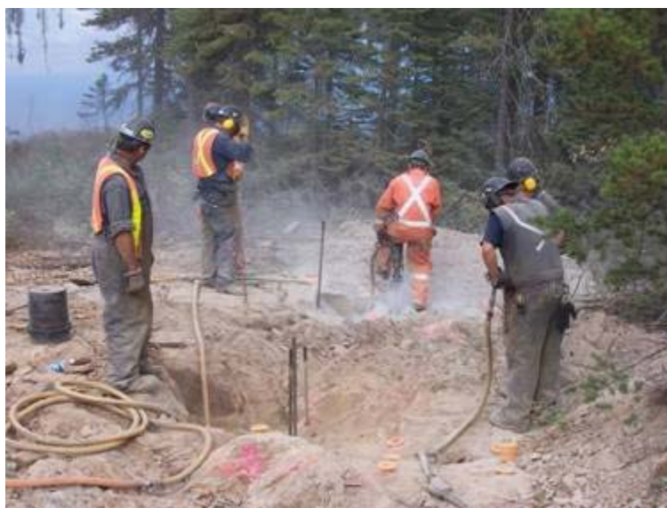
Picture of workers preparing stripped outcrop site #1 for blasting.
